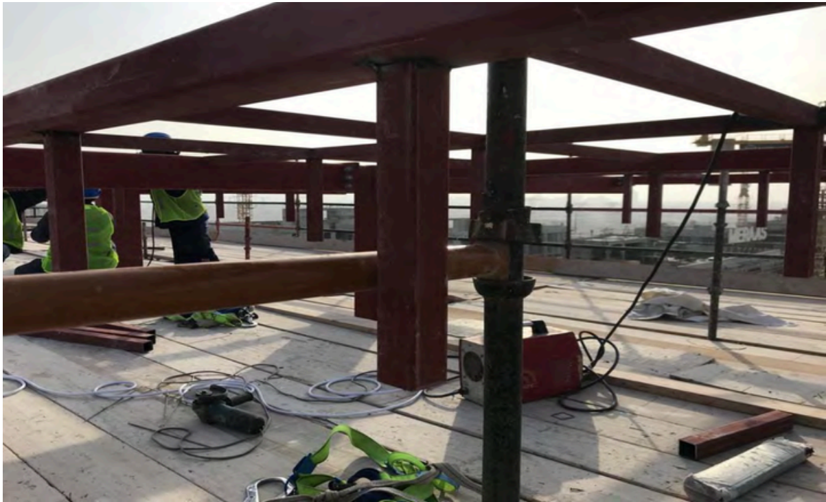
ROOF CANOPY STRUCTURE – SOBHA DUBAI HILLS
