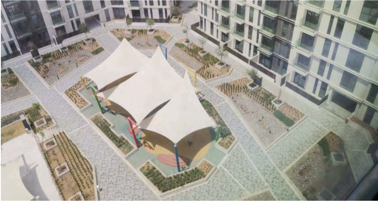
SHADE STRUCTURE AT EXPO 2020 PARCELS
