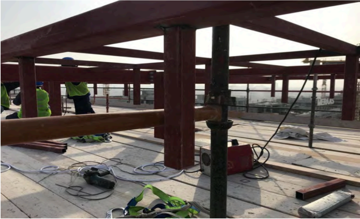
ROOF CANOPY STRUCTURE – SOBHA DUBAI HILLS
