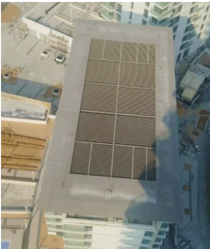
FIBREX CONTRACTING LLC The Cove II" Proposed Mixed Use Development Roof Canopy Steel Structure with ACP Cladding
