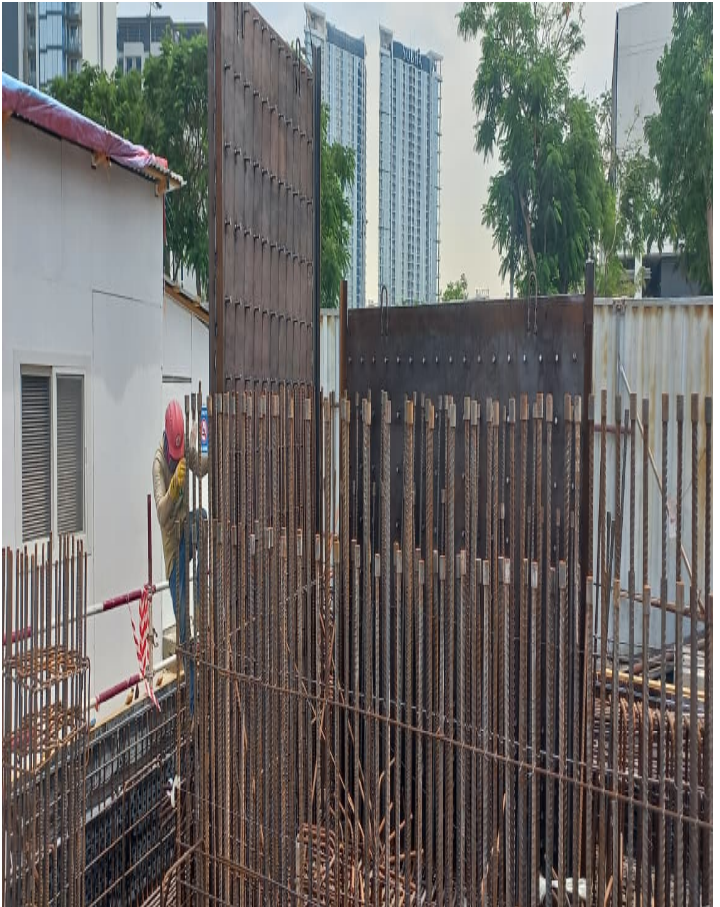
Shear Stud with Coupler Welding
