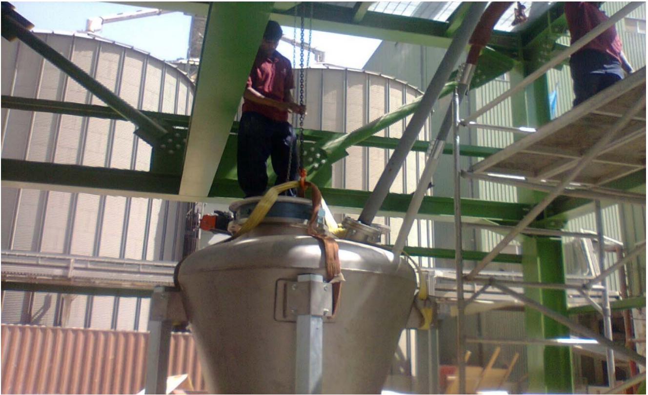
Figure 18:- S S Sender Vessel Erection Work & Piping at IFFCO, Sharjah.
