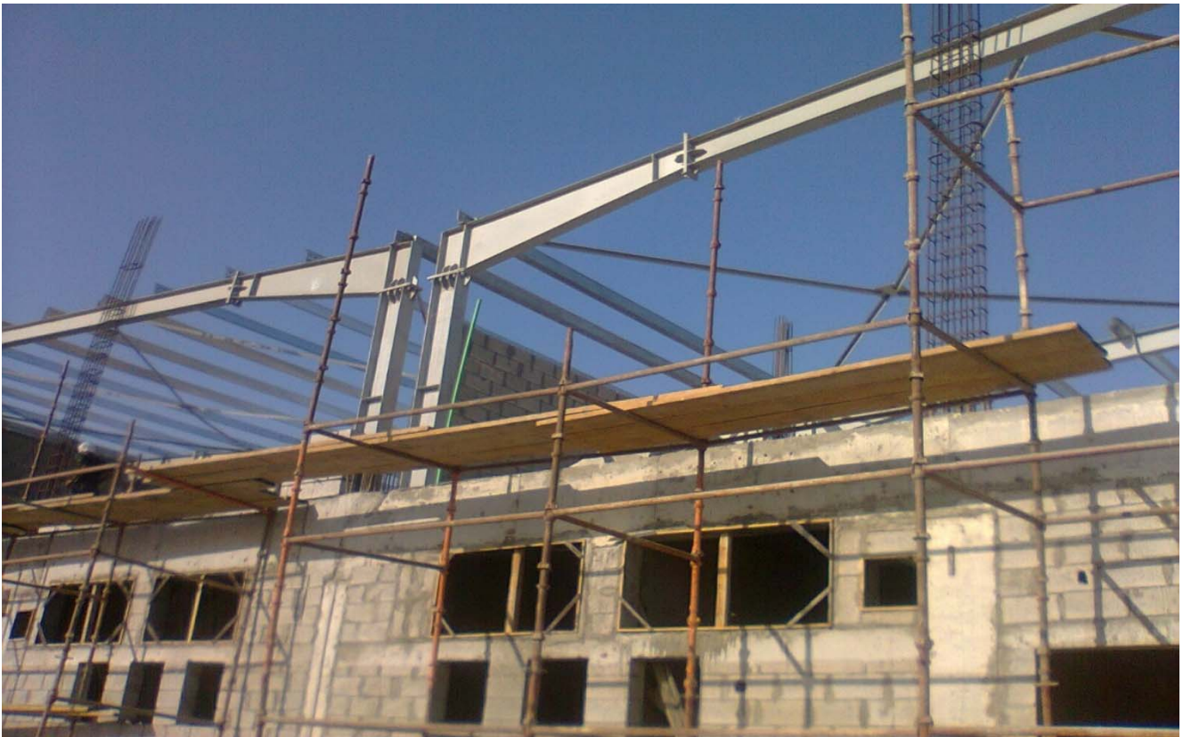
Figure 19:- Roof Structure & Erection Work of Warehouse
