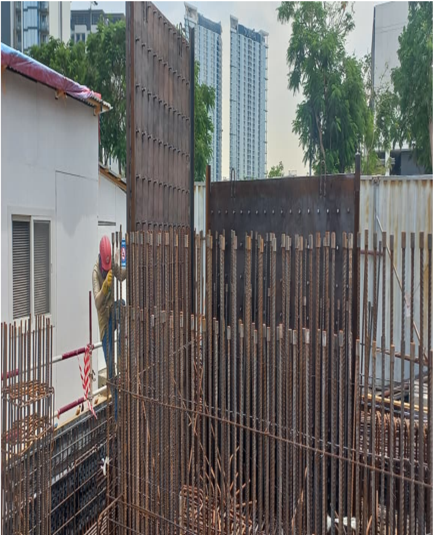
Shear Stud with Coupler Welding
