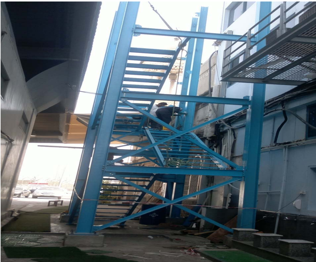
Figure 25:- Additional Stucture Staircase at Emigrain, Sharjah Khalid Port
